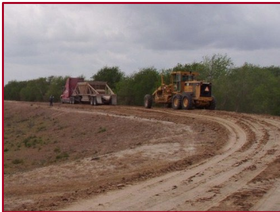
Lower Rio Grande Levee
