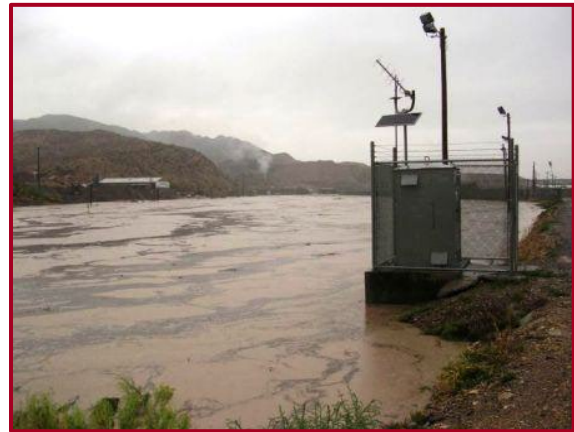
Rio Grande Gaging Station
