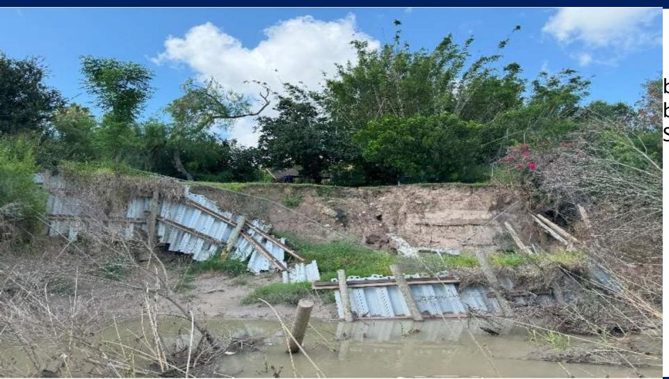
Failed vinyl sheet pile bulkhead along the bank of the Arroyo in Segment 2
