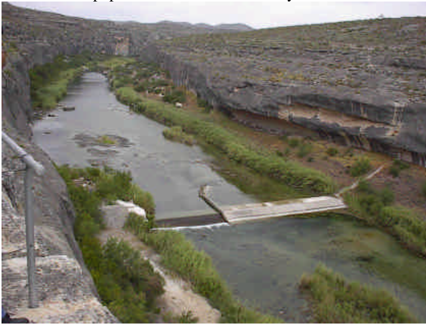
Figure 15. The Pecos River at the USIBWC Langtry gage site.
