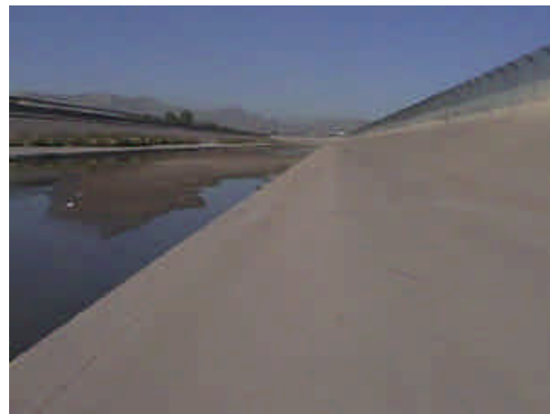
Figure 26. Channelized Section in Segment 2308.
