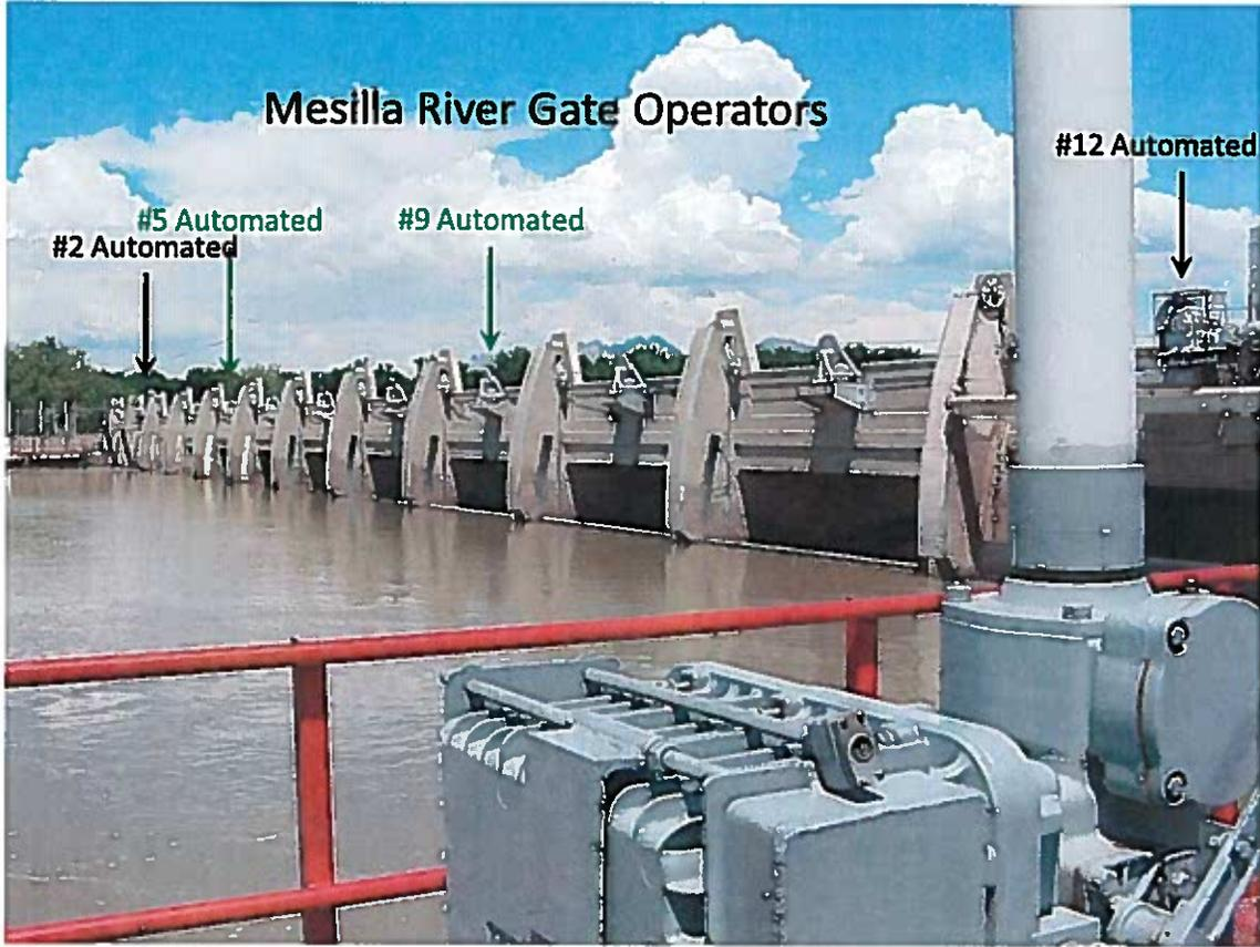
Figure 9. Photograph of Mesilla Dam showing gates currently automated and proposed for automation
