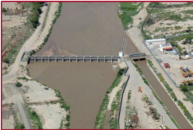
American Diversion Dam
