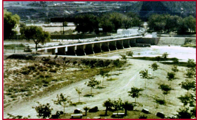
American Diversion Dam
