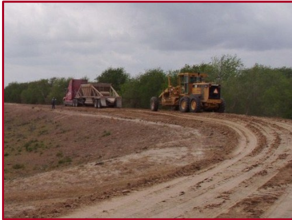
Lower Rio Grande Levee
