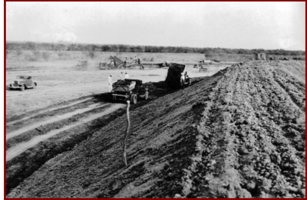
Lower Rio Grande U.S. Main Floodway
