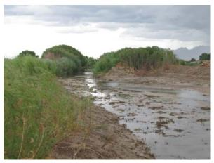
Photo 17: River mile 36. MxIBWC completed dredging operations. Note dense vegetation (primarily salt cedar) along Rio Grande downstream of dredging operations, and widening of main channel.
