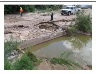
Photo 39: River mile 77.5. Broken Box Culvert Drain.
