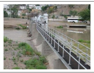
Photo 6: River mile 1.5. International dam, looking to Mexico. Note culvert upstream of International Dam for transfer of water to Mexico.
