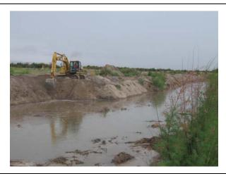
Photo 21: River mile 48-50. MxIBWD dredging operations; note bank cut back of at least 10 feet, and bank vegetation removal.
