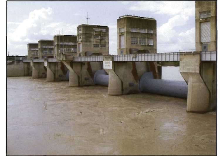
High water at Anzalduas Diversion Dam
