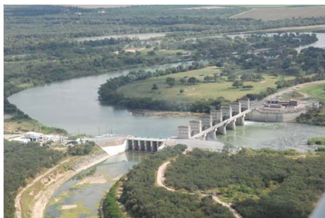
The Commission performed routine maintenance on the gates of Anzalduas Dam.
