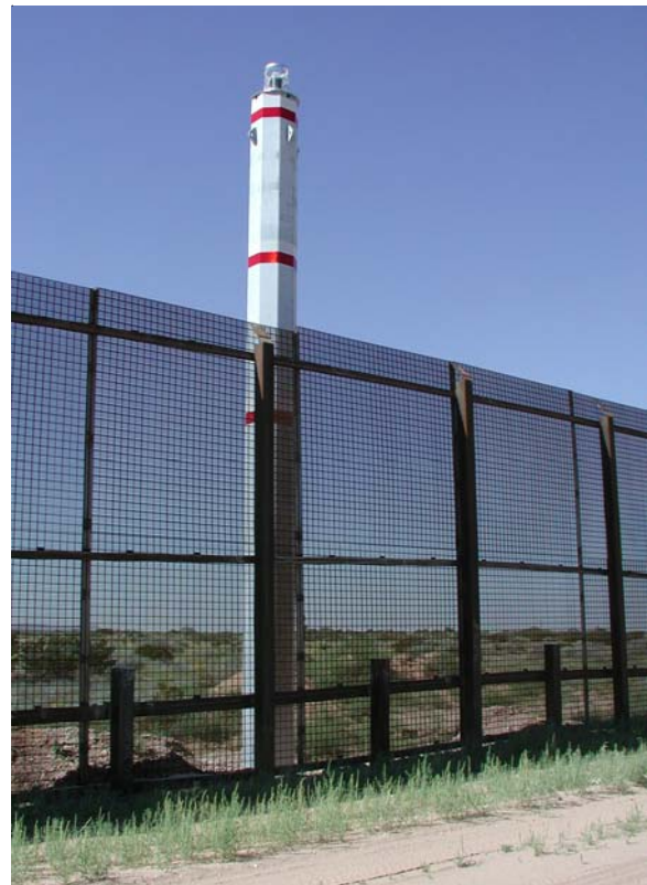
New boundary markers were installed as part of a pilot project near El Paso, Texas-Ciudad Juarez, Chihuahua.
