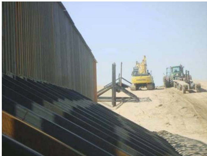
Construction of the border fence along the international land boundary.
