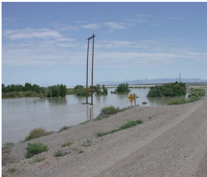
Rio Grande levees near the Presidio-Ojinaga International Bridge were put to the test in both countries.
