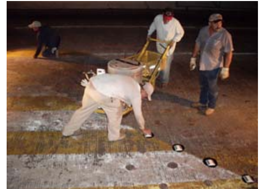
The Commission demarcates the boundary on the bridges at night to minimize traffic disruption.
