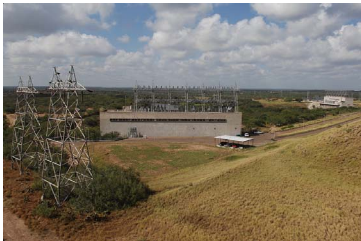
The Commission is considering installing a low-flow generating unit at the Falcon Dam Power Plant.
