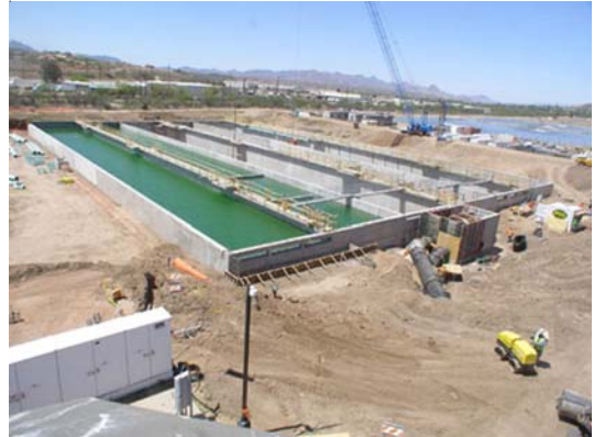
Construction of the NIWTP upgrade.
