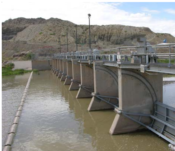
Three of American Dam's gates were replaced during 2008.
