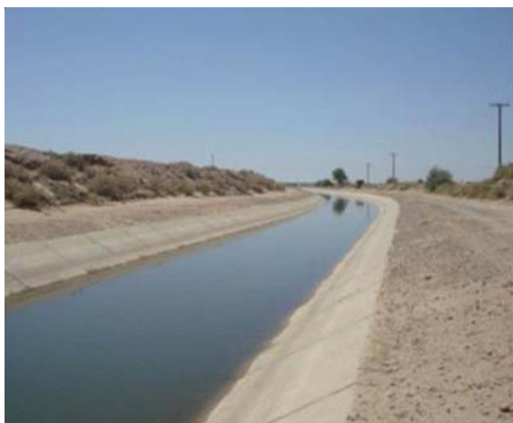
The Wellton-Mohawk Drain after sediment was removed.
