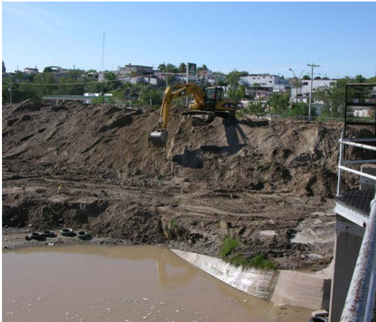
The Commission removed sediment at El Paso-Ciudad Juarez in accordance with Minute 313.
