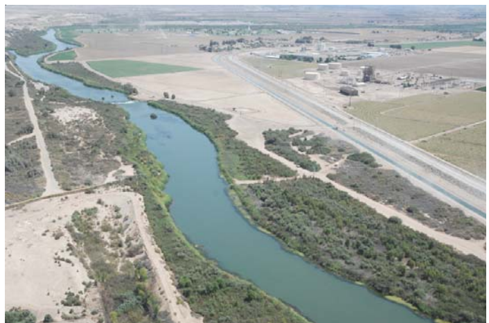
The Colorado River at the Northerly International Boundary, Yuma Desalting Plant at top right.
