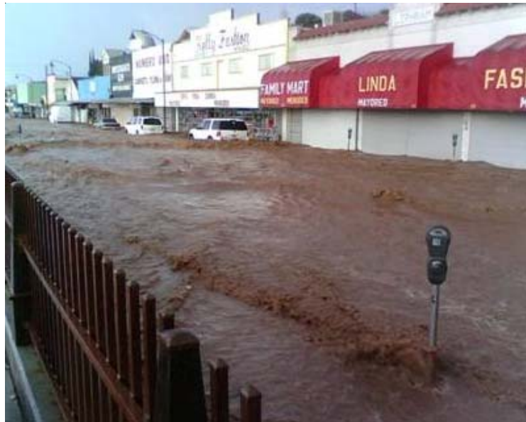
Flood in Nogales, Sonora that caused the collapse of part of the Nogales Wash tunnel.
