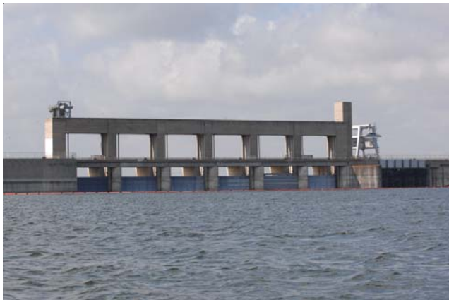
Falcon Dam experienced normal conditions for most of the year.
