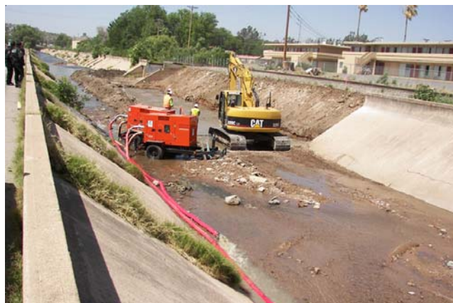
Repairs were made to the Nogales Wash before the rainy season.
