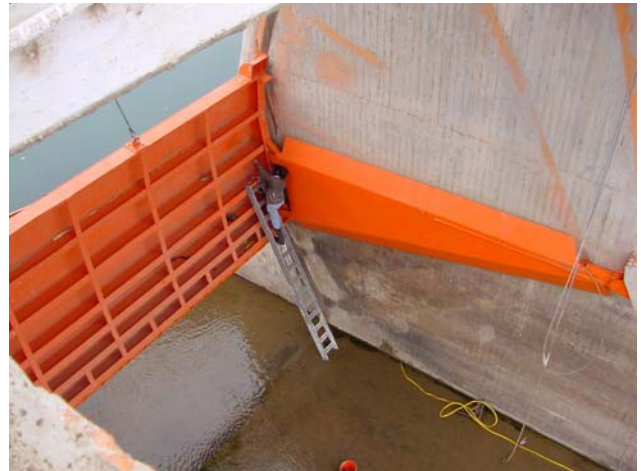
Morelos Dam maintenance
