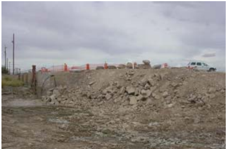
Work at Riverside Dam
