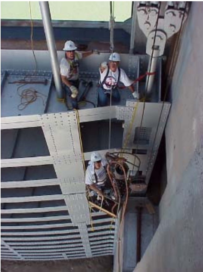
Falcon Dam spillway gate
