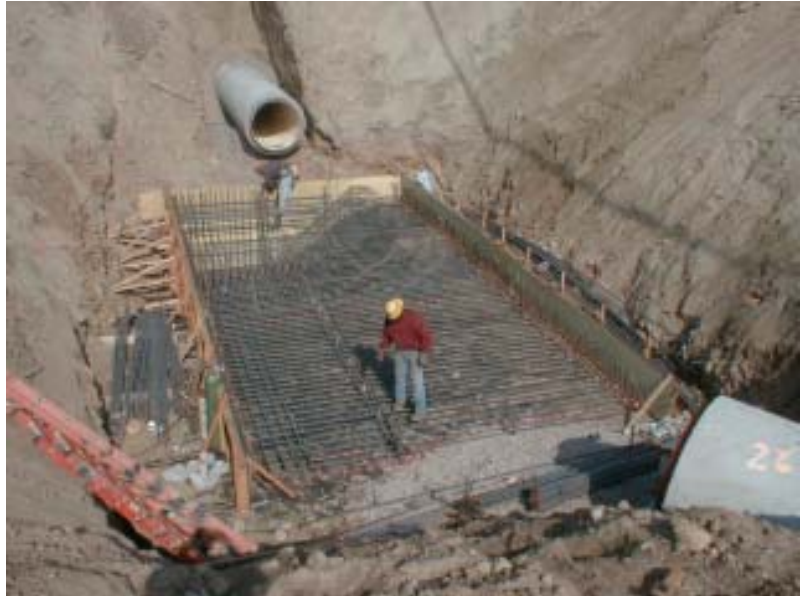
Work on the Primary Effluent Return Connection
