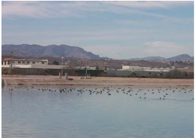
Nogales International Wastewater Treatment Plant
