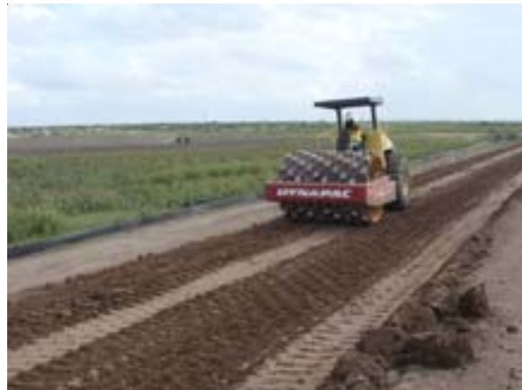
Construction is progressing on Lower Rio Grande Flood Control Project levees.
